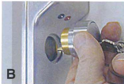
B. Remove old cylinder and Insert new cylinder.
